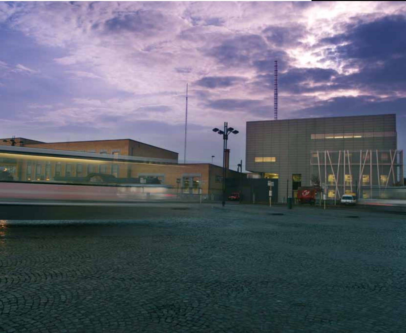
Seinhuis, Brugge (B) | Architect: Eurostation (B) | Limeparts: Quartz-Zinc®
